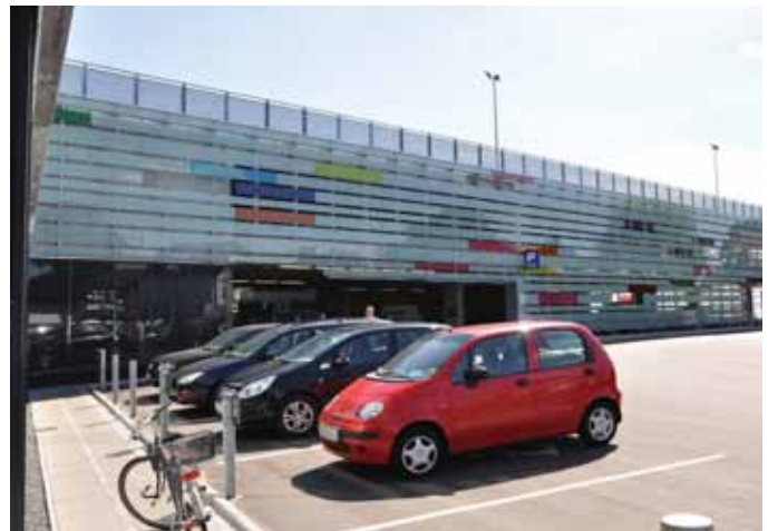
Multi-storey car park, shopping mall Nørreport Centeret, Holstebro, Denmark
