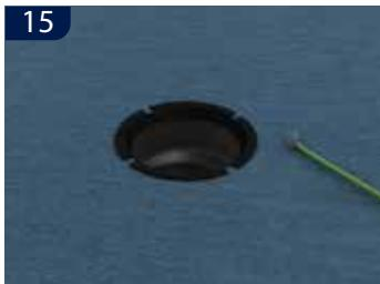
**(UK)** If an equipotential bond is required, connect the earth electrode to the earthing screw at the upper edge of the membrane flange.
