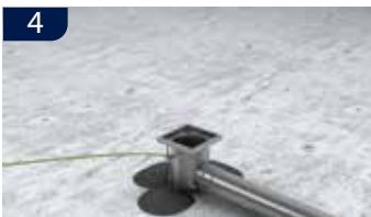
**(UK)** To make sure that the drain will not float up during casting, it is recommended that the feet of the adjustable legs are set in concrete. If equipotential bonding is required, connect the earth wire to one of the adjustable legs.
