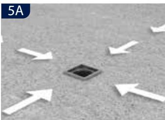
**(UK)** Cast the floor with the recommended fall towards the drain. For drains with 50 mm liquid membrane flange, a liquid membrane can be applied in accordance with the guidelines of the supplier of the liquid membrane. Lay the tiles or apply epoxy.
