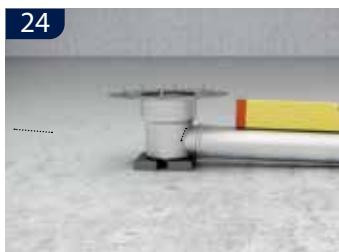
**UK** Adjust the lower part to the correct height and adjust the flange to make sure it is level. Install the drainage pipe with correct fall according to applicable regulations.
