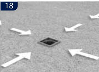
**UK** Cast the floor with the recommended fall towards the drain. For drains with 50 mm liquid membrane flange, a liquid membrane can be applied in accordance with the guidelines of the supplier of the liquid membrane
