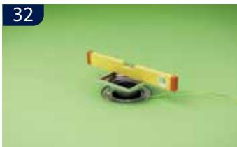
**UK** Adjust the upper part to the correct height and make sure it is level. BLÜCHER recommends using the 4 adjustment screws to ensure that the upper part is 100% level.
