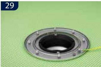
**UK** For a tight solution center the upper part over the lower part, place the sealing ring directly into the lower part. Ensuring the sealing ring is placed the correct way up. Fix the clamping ring with uniform torque. If an equipotential bond is required, connect the earth wire to the earthing screw at the upper edge of the membrane flange.
