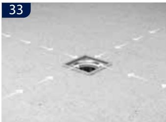
**UK** Cast the floor with the recommended fall towards the drain. For drains with 50 mm liquid membrane flange, a liquid membrane can be applied in accordance with the guidelines of the supplier of the liquid membrane. Lay the tiles.
